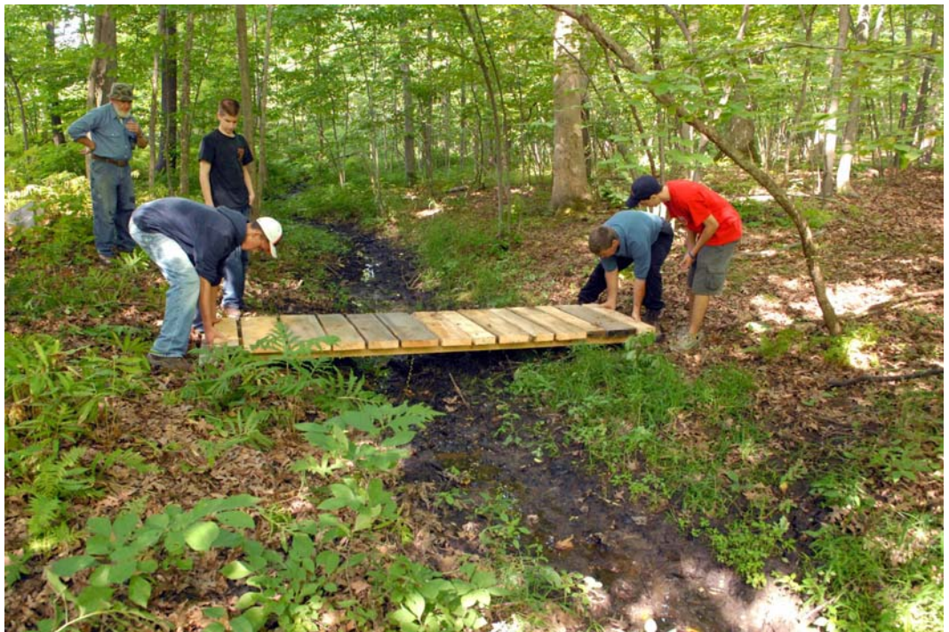
A bridge-building project nears completion at the Swift Preserve
